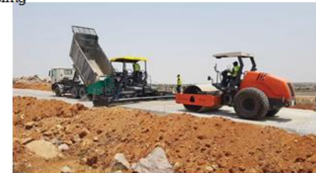
Utilization of Industrial waste in road construction
