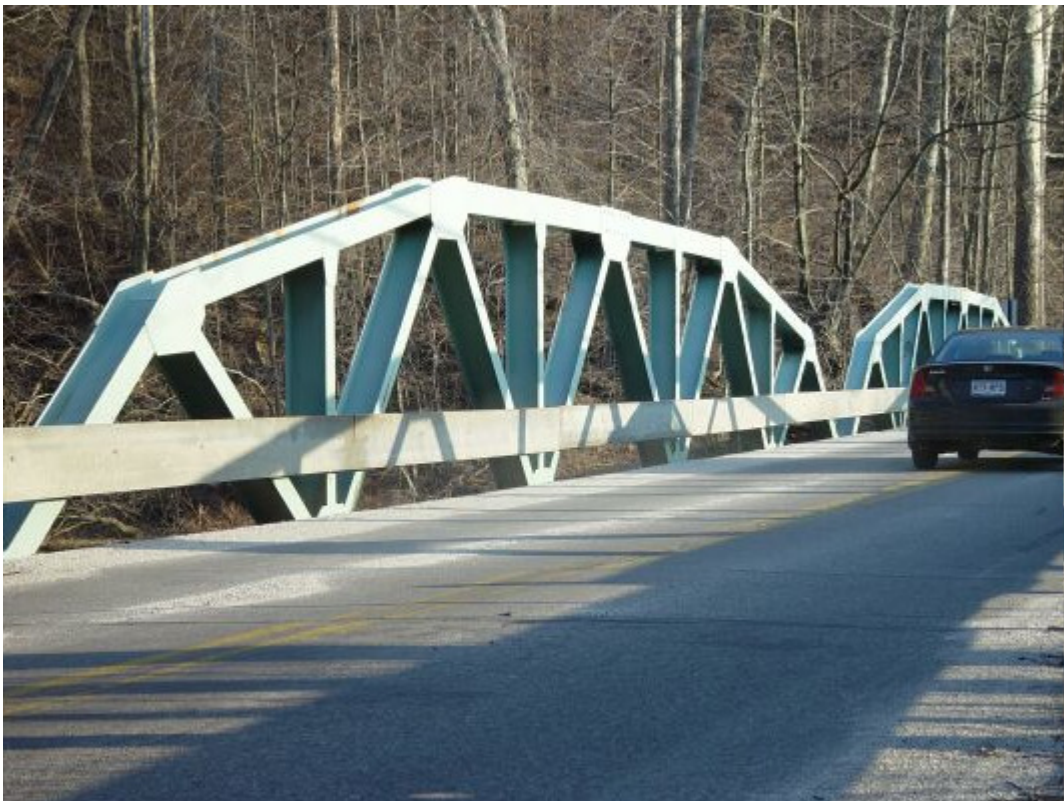
Bridge truss— plane truss
