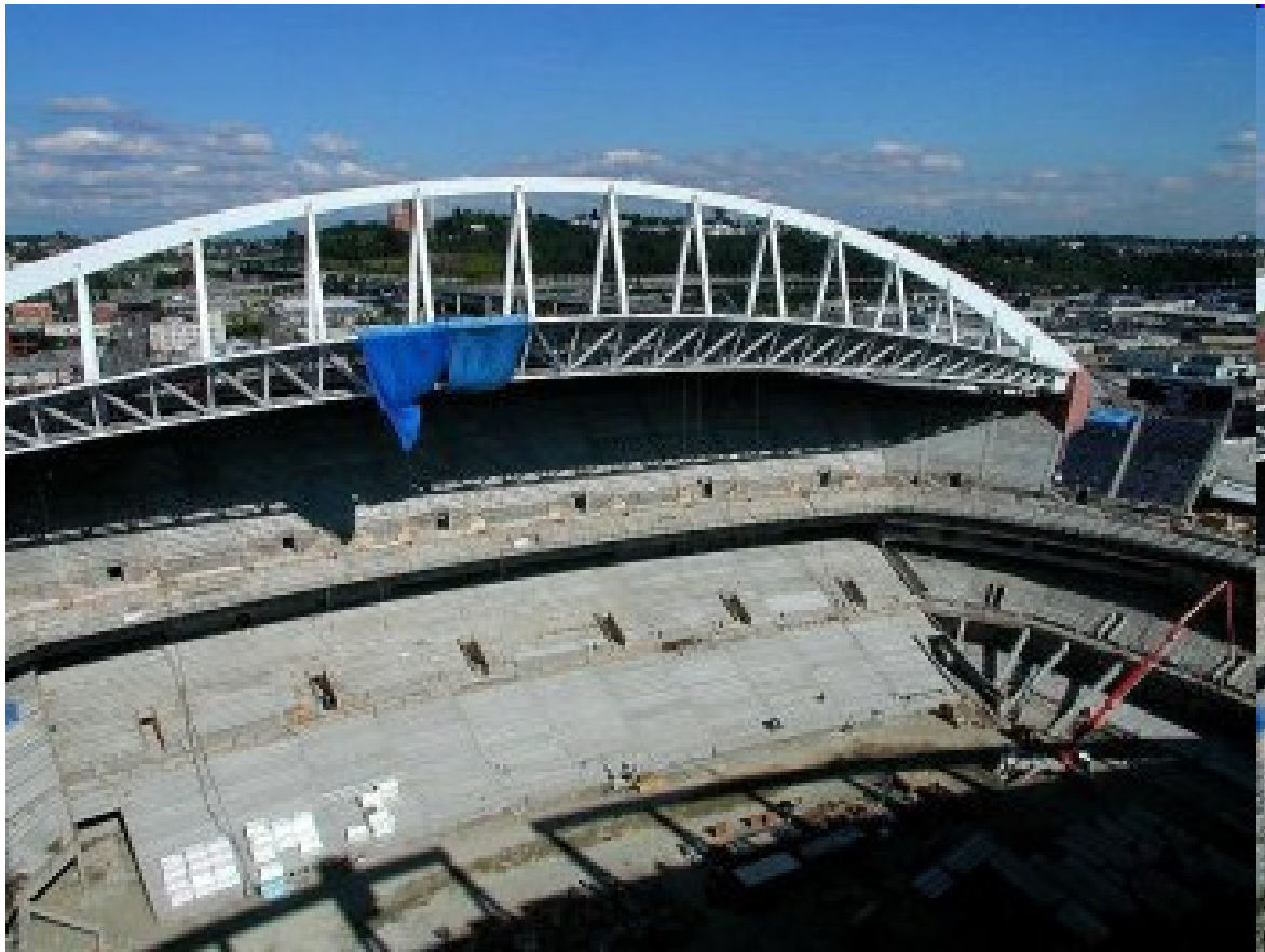
Truss for stadium
