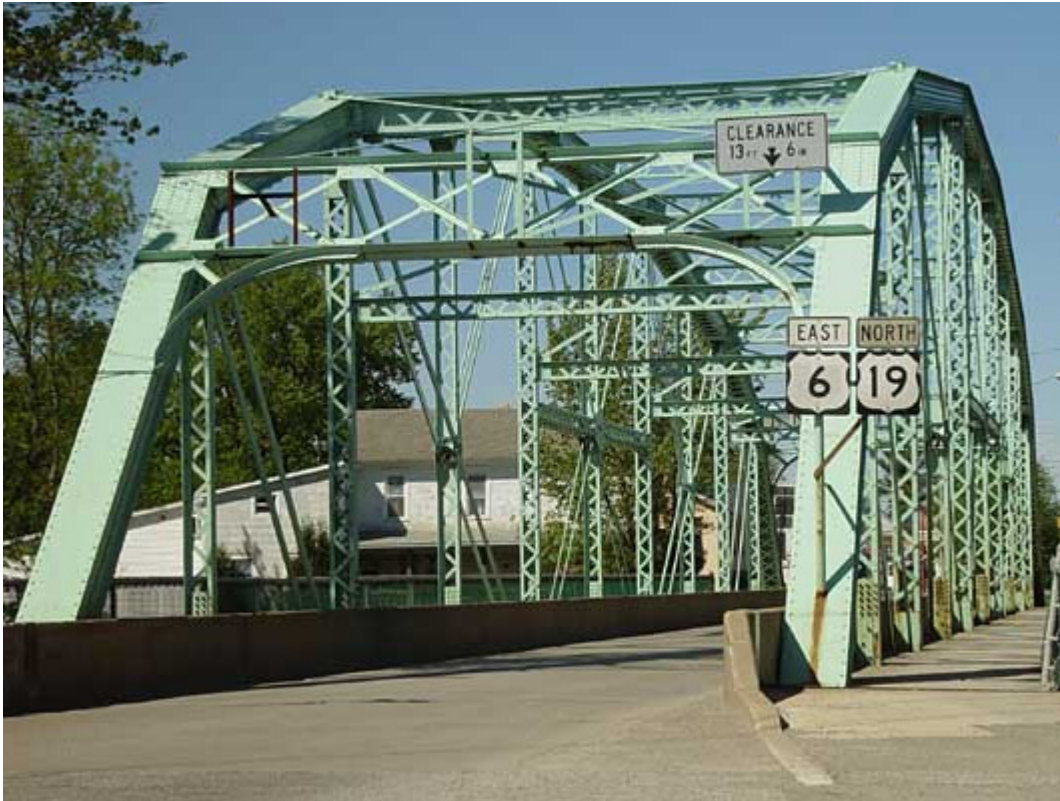
A bridge truss
