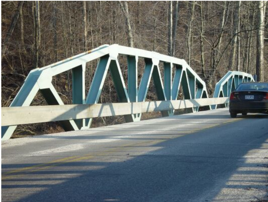
Bridge truss—plane truss
