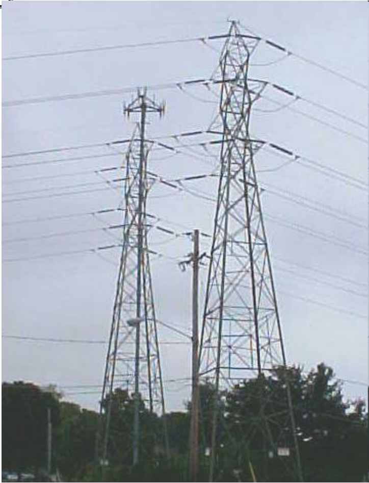
Transmission line tower— space truss
